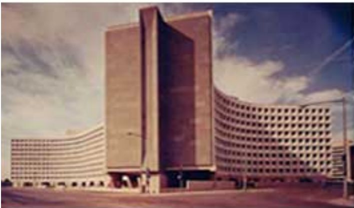
H.U.D. Building Washington 1968
