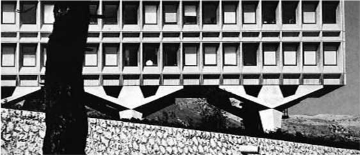
IBM Research Center in La Gaude (France), 1960-62
